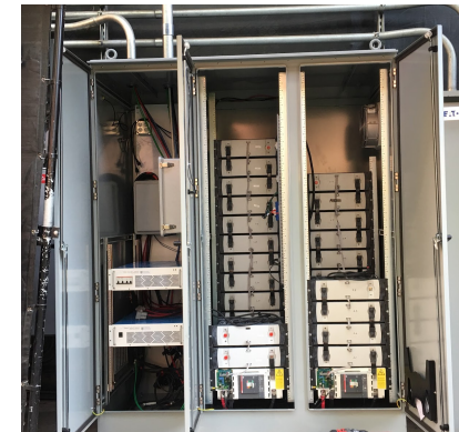
56 kWh Saft BESS in PS 9
