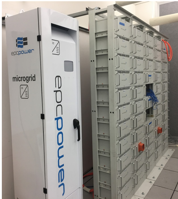
Microvast Li-ion Battery with EPC Power Inverter
