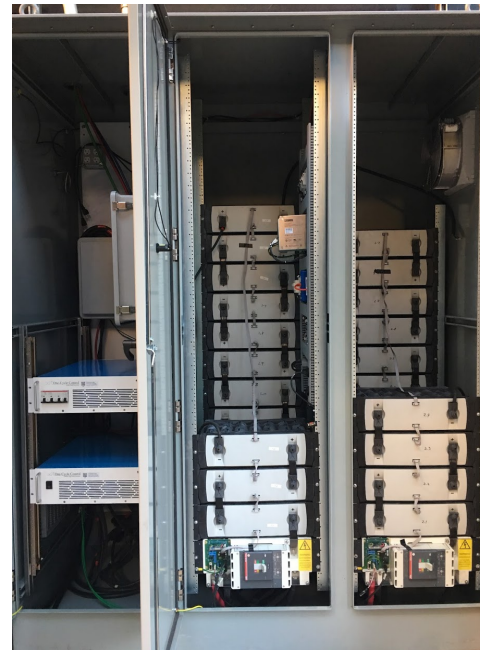
Saft Li-ion Battery with OCC Inverters
