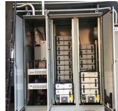
56 kWh Saft BESS in PS 9
