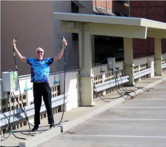
Level 2 Smart Chargers with circuit sharing among 4 connected EVs
