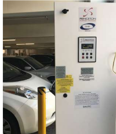
Princeton Power CA 30 V2G DCFC with Nissan Leaf
