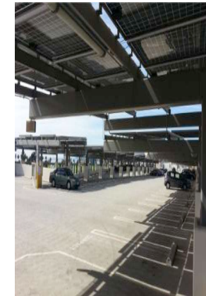
213 kW PV With PMU/PQA
