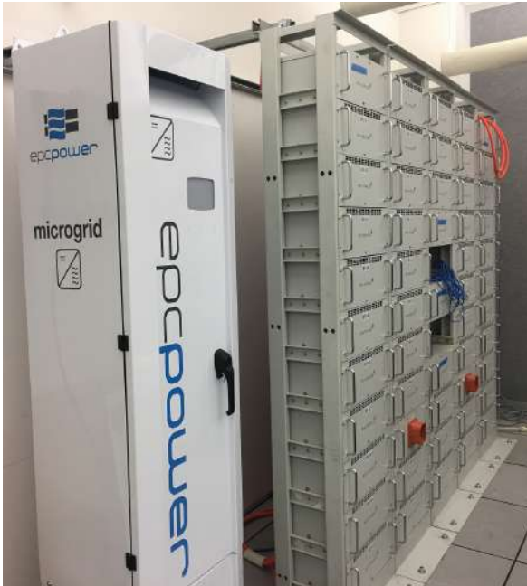
Microvast Li-ion Battery with EPC Power Inverter
