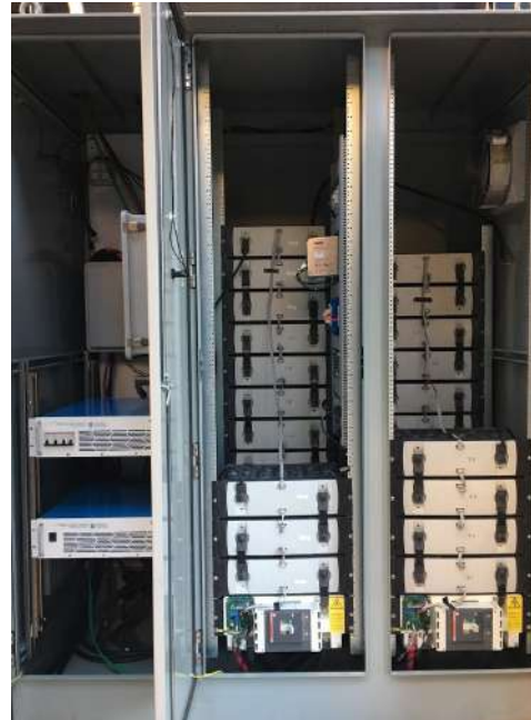
Saft Li-ion Battery with OCC Inverters
