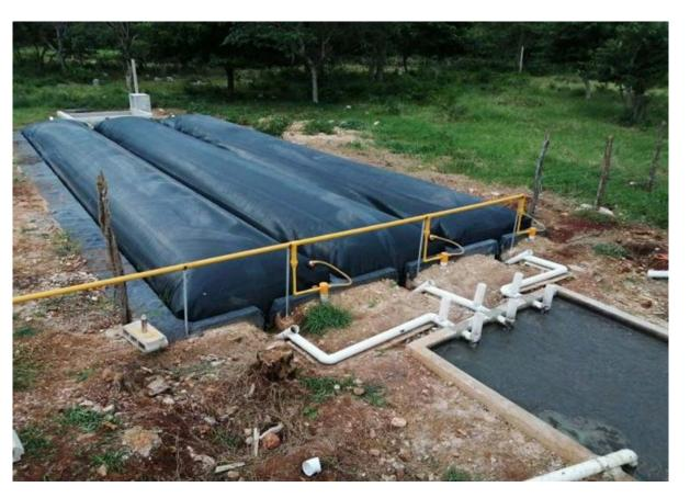
Biodigester (source of biogas)
