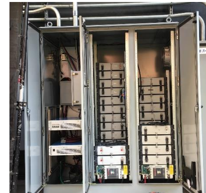
56 kWh Saft BESS in PS 9
