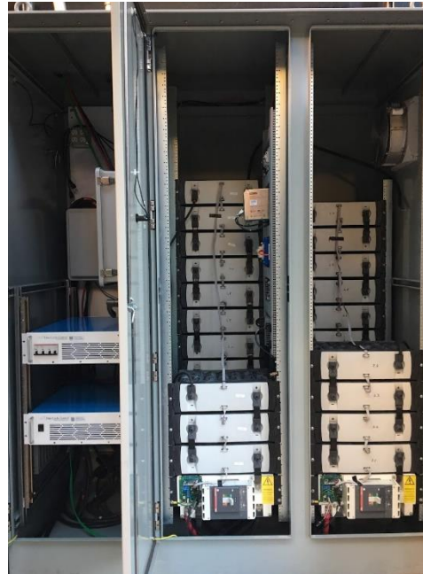
Saft Li-ion Battery with OCC Inverters
