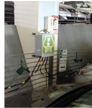
14 level 2 smart EV charging stations
