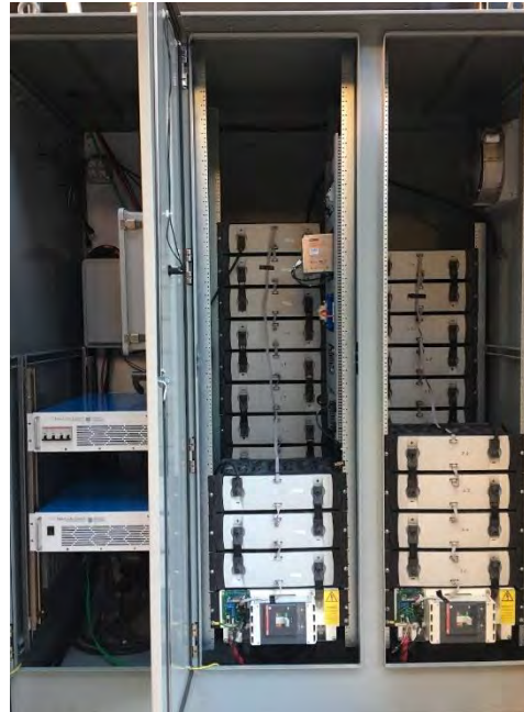
Saft Li-ion Battery with OCC Inverters
