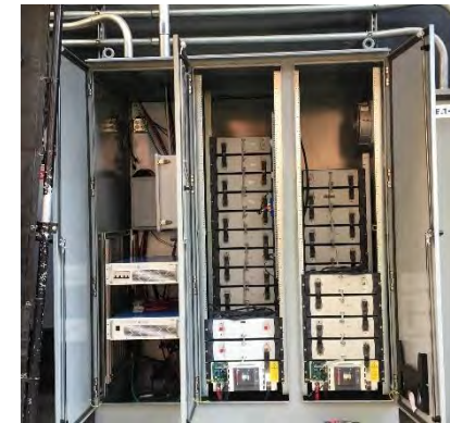
56 kWh Saft BESS in PS 9
