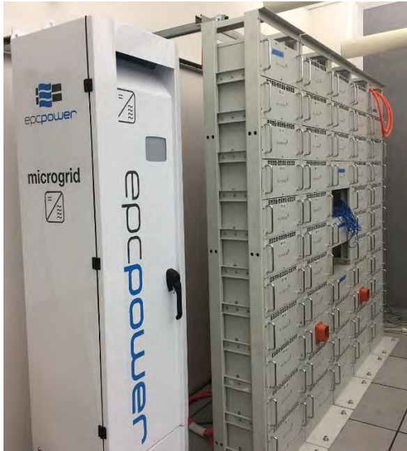
Microvast Li-ion Battery with EPC Power Inverter
