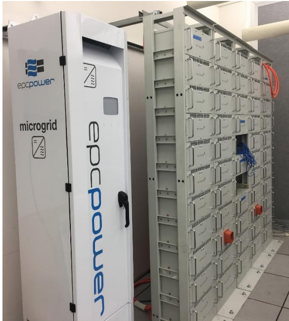
Microvast Li-ion Battery with EPC Power Inverter
