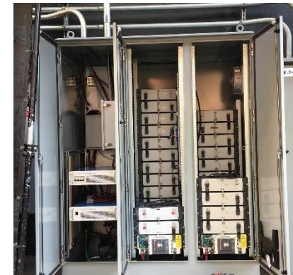
56 kWh Saft BESS in PS 9
