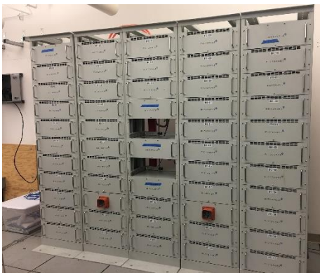
50 kWh Microvast Li-ion Battery with EPC Power inverter
