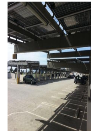
213 kW PV With PMU/PQA
